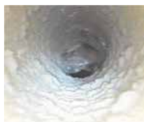
Dirty supply air duct in a hospital
